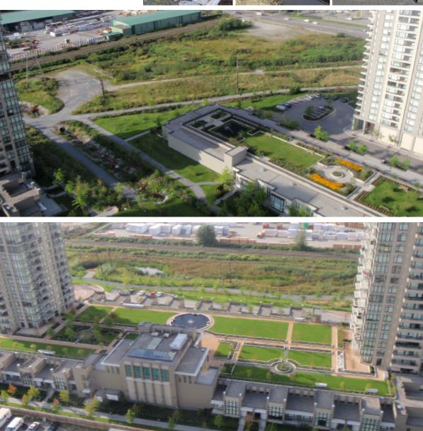
In this project a series of residential towers required a design solution that would allow for safe collection and disposal of storm water from all paved and roofed areas of the site into the adjacent, sensitive fish-habitat creek. After an extensive environmental impact assessment, the design solution provides for a series of bio-filtration ponds and that allow for the required storm water purifying process. In addition, the newly created natural buffer created a wildlife and bird habitat.
